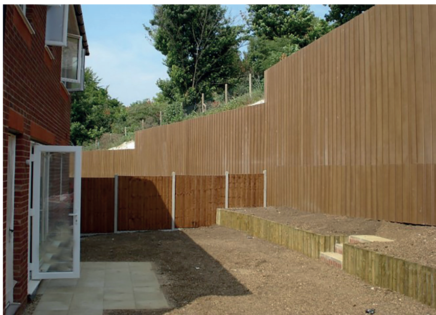
A King post wall after construction (above) and with cladding installed by others (below).
